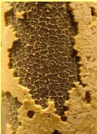
Limescale in the heat exchanger
