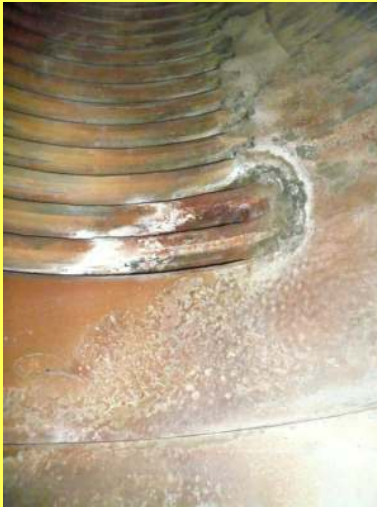
Lime precipitation in the boiler
